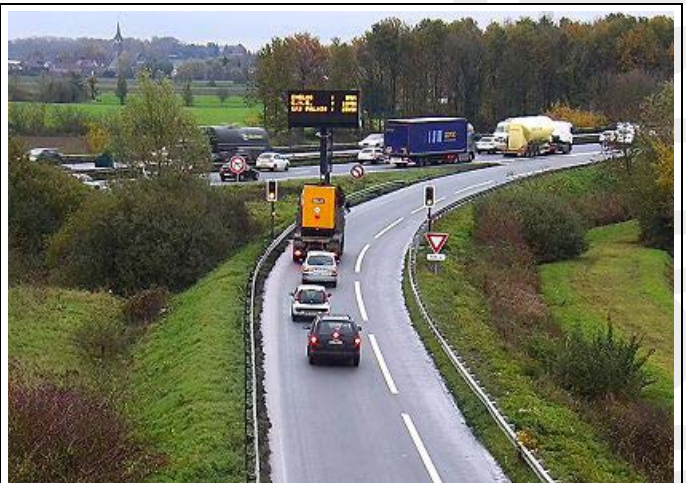
©DIR Nord – Ramp metering on junction n°8 Dunkerque->Lille
