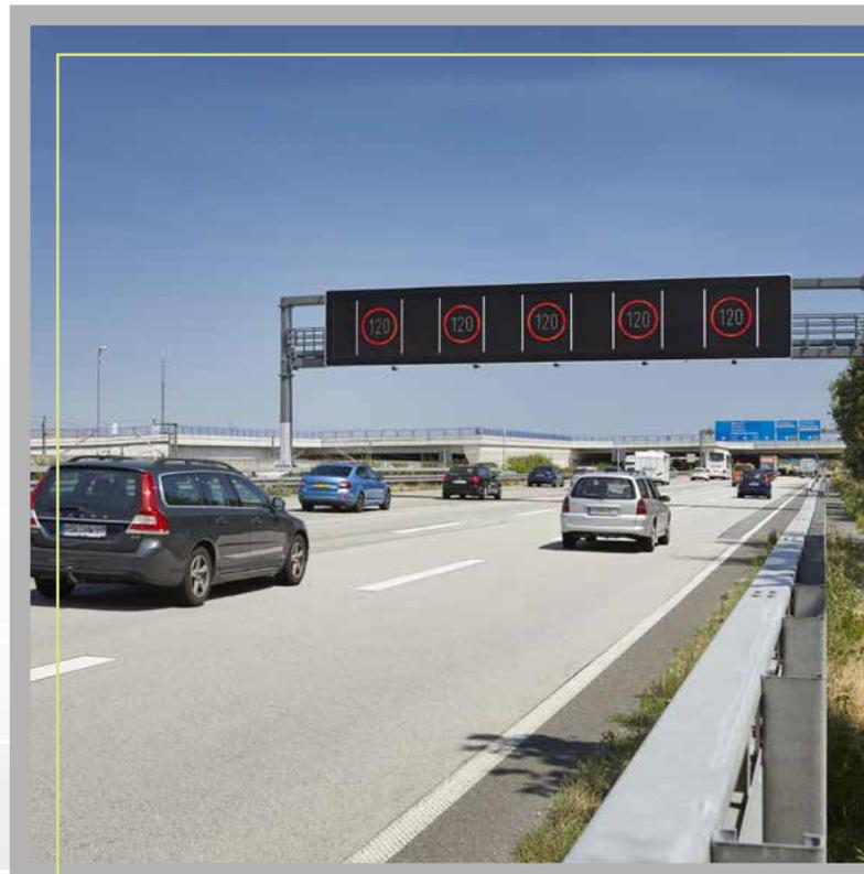
The system also serves to protect roadworks and broken down vehicles and to warn of adverse weather conditions.
